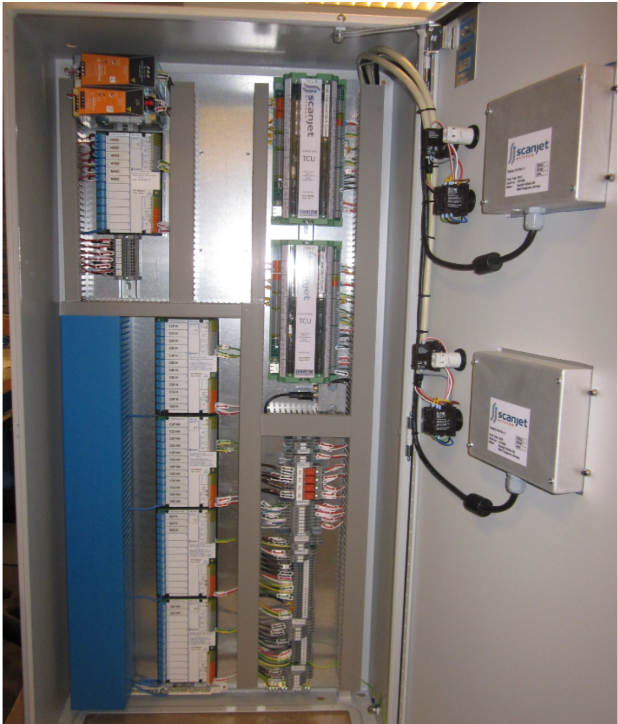
Example of one system cabinet
